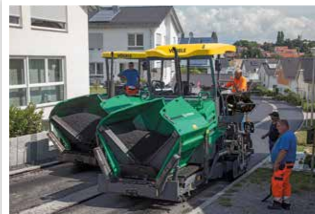
PAVEMENT REHABILITATION ON ACCESS ROADS
