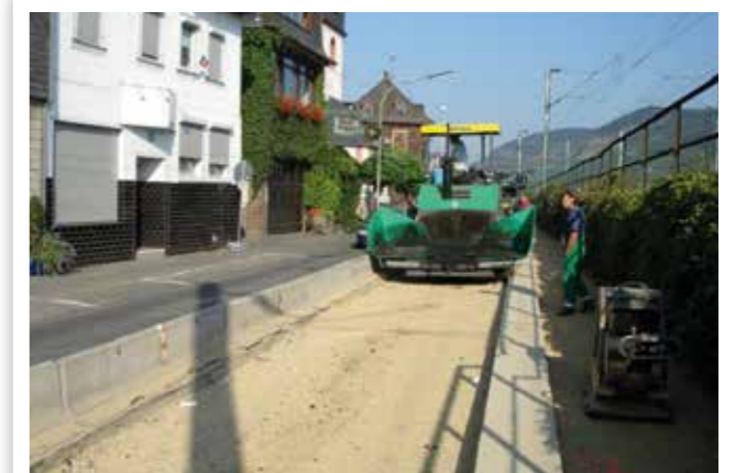
PAVEMENT REHABILITATION ON MUNICIPAL ROADS
