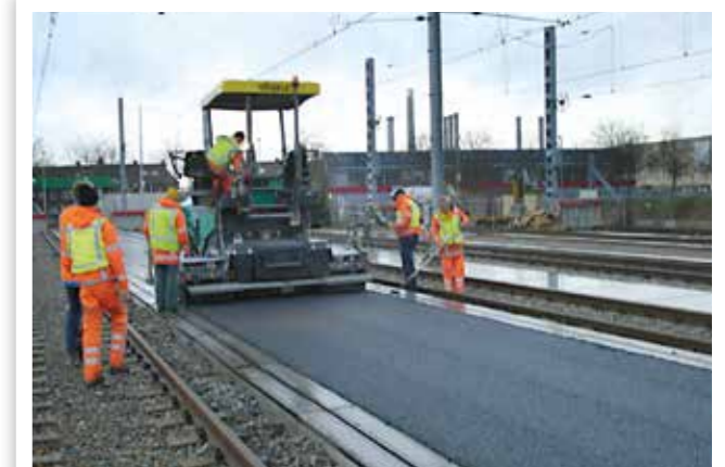
ASPHALT PAVING ON RAILWAY PLATFORMS
