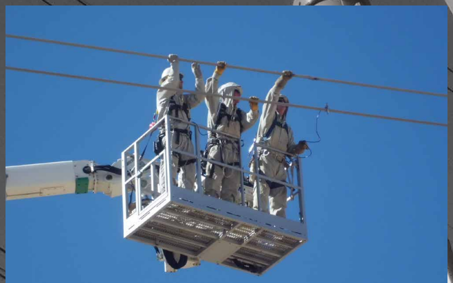
Boom Leakage Detector indicates the actual current experienced by the platform personnel and FRP boom.
